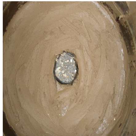
(b) Installed column
