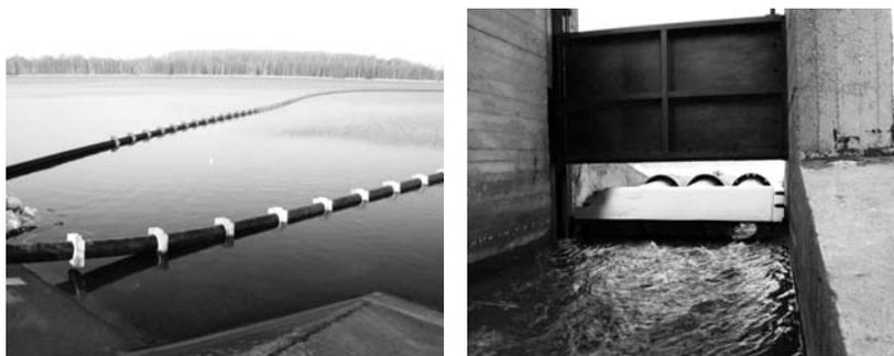
Fig. 2. Hypolimnion discharge channel with the Olszewski tubes
