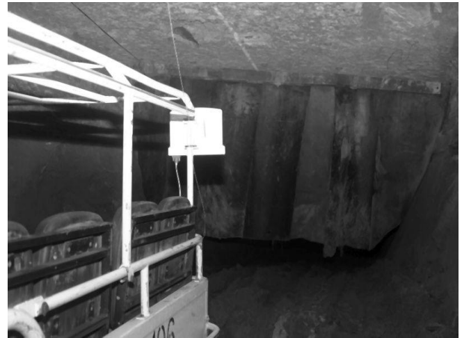
Fig. 12. Rubber curtain to control air circulation
