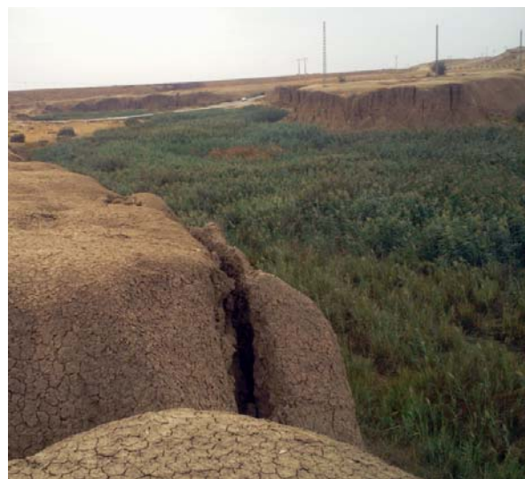
Fig. 5. Banks erosion of the Chellif wadi; photo: B. Remini
