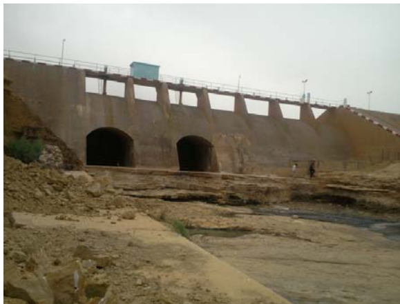
Fig. 3. An overview of the Boughezoul dam; photo: B. Remini
