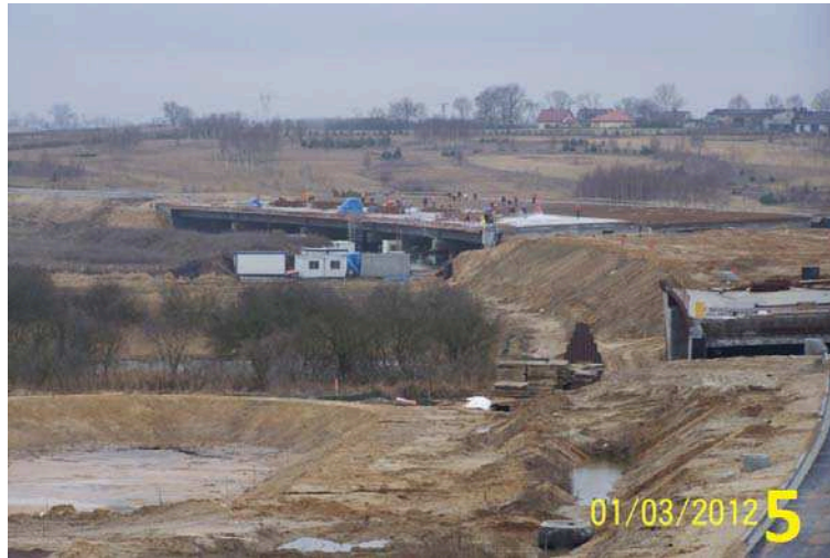
Photo 5. Construction of flyovers in Natura 2000 Samica Valley [02.03.2012, http://www.s11-zlotkowo-rokietnica.pl ]
