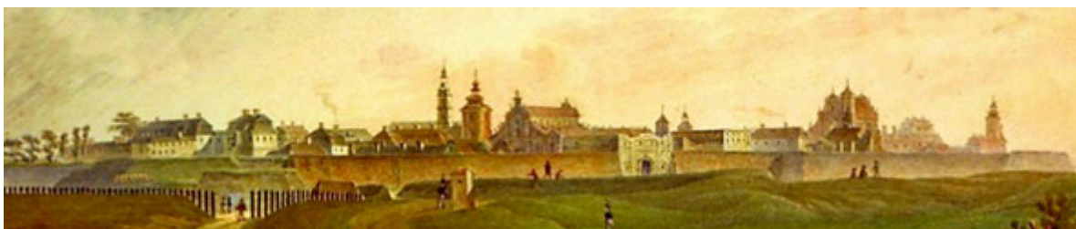
7. Padua, maintenance of walls, state of 2015 year
