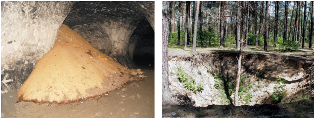
Fig. 6. Caving-in underground the Nagórzyckie Grottos and the subsidence on the surface
