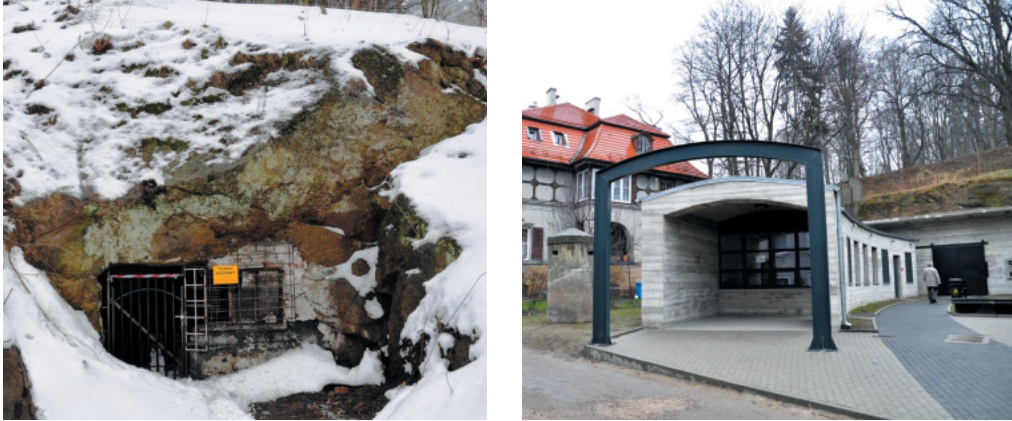
Fig. 9. Tunnel in the Park Mountain in Kamienna Góra- before the restoration work and the entrance to the underground tourist passage
